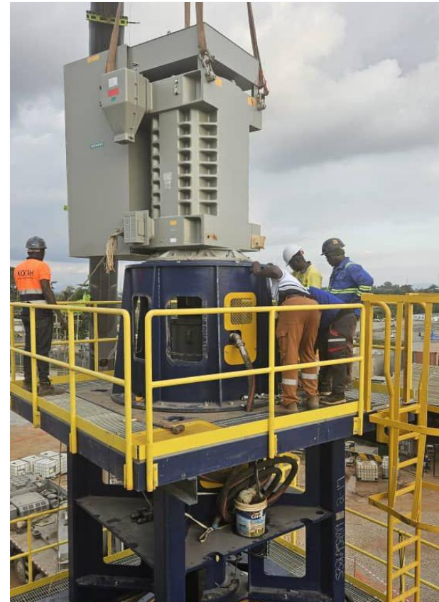
VXP Mill Package Installation
