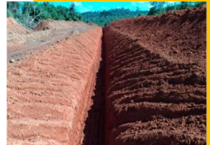
Trenching at the Baldo zone, Cajueiro project
