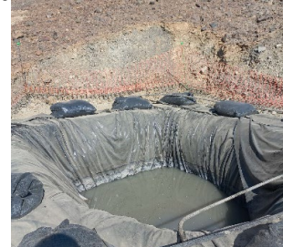
Minimizing our environmental footprint and protecting+preserving land+water by using membranes to protect against drill-site spills and to recover-recycle used water as well as protecting indigenous plant species.
