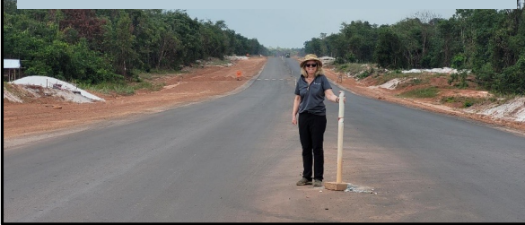
Road widening and paving underway to within 10 km of Omai property
