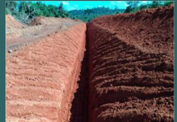
Trenching at the Baldo zone, Cajueiro project
