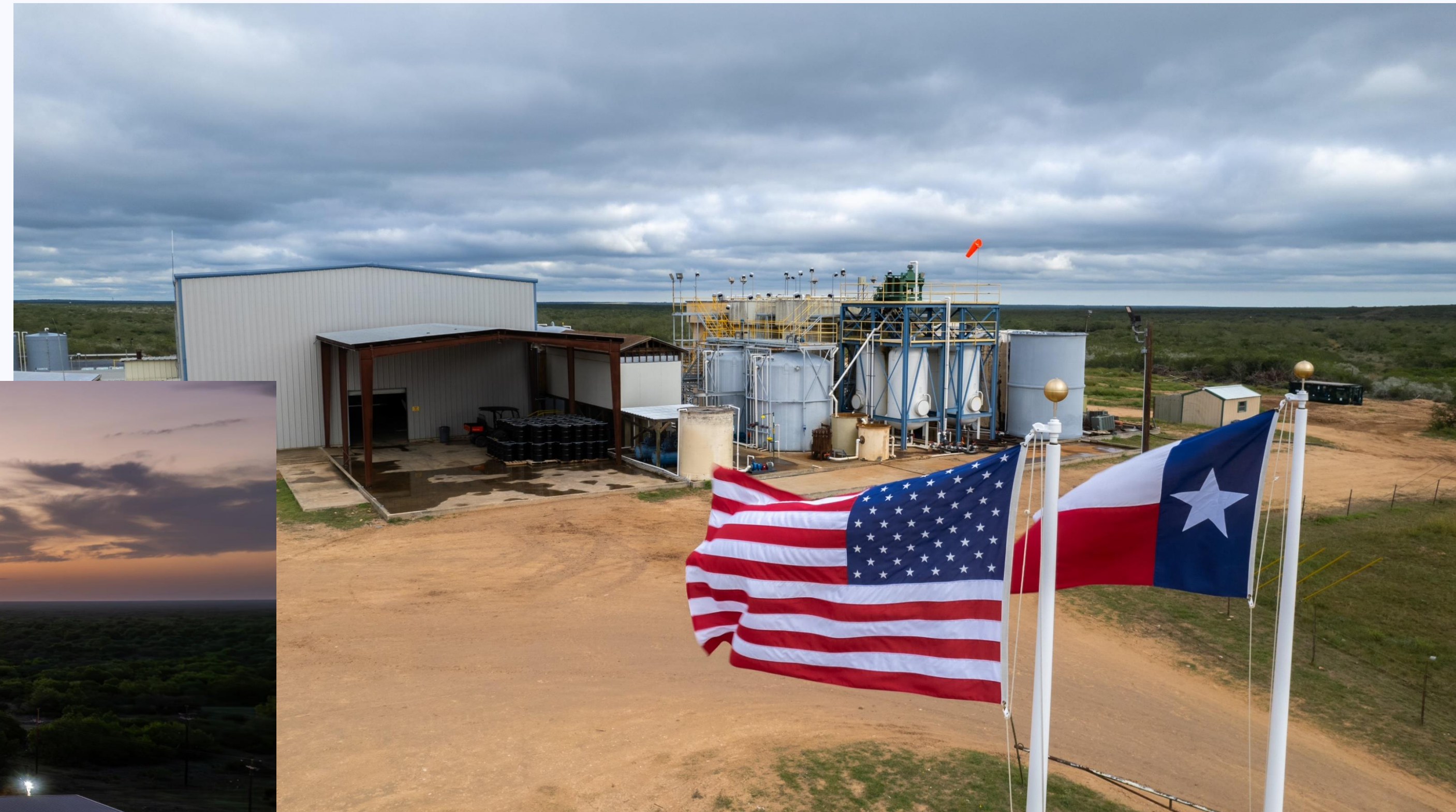
Rosita ISR Uranium Central Processing Plant: in production as of 11/23
