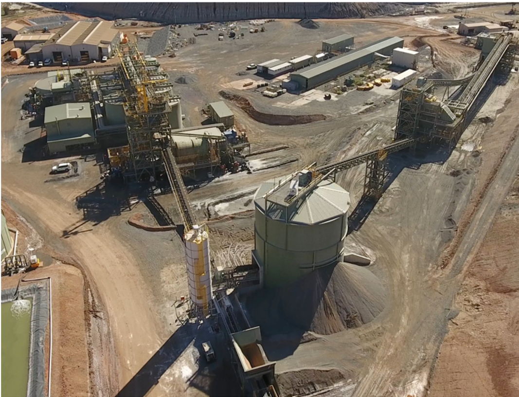
Norseman processing plant comfortably operating at 1.2Mt per annum
