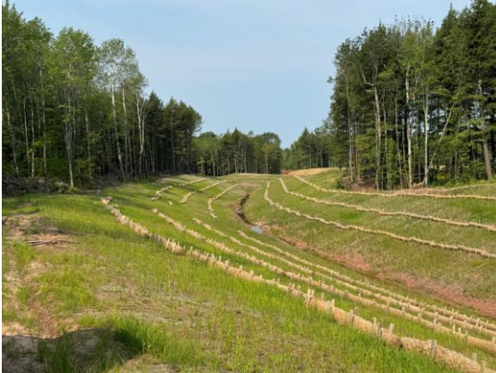
Stream Diversion Structure
