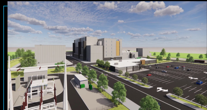
EcoProBM, SK On and Ford are planning to invest C$1.2 billion to build a cathode manufacturing facility in Bécancour, Québec.
