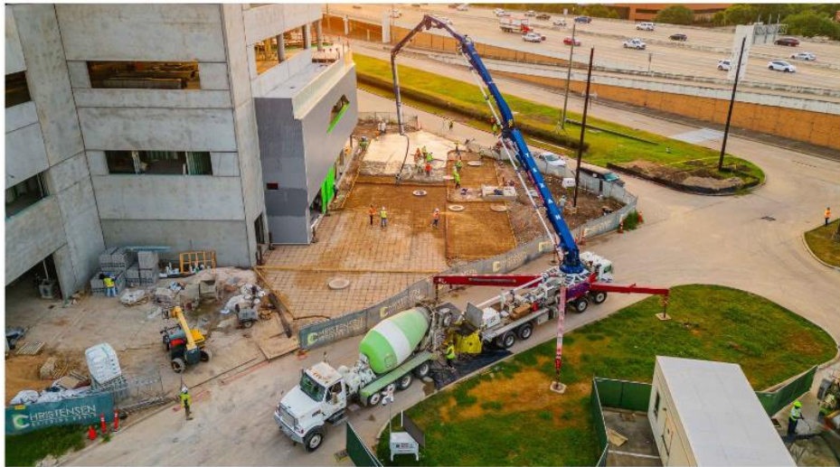
OPUS SCM concrete for the Porsche Sugar Land pour batched, placed, and finished like conventional mixes.
