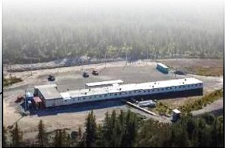
Initial Construction Starter Camp *installed septic
