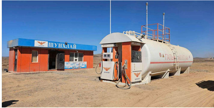
Temporary Fuel Station
