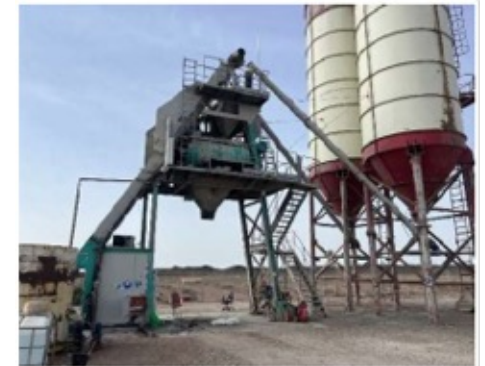
Concrete Batch Plant Establishment
