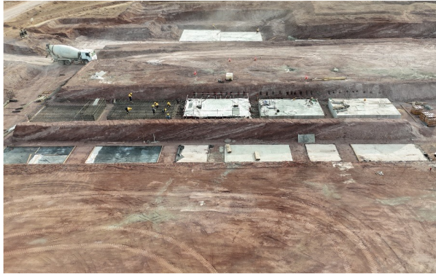
Process Plant Footings
