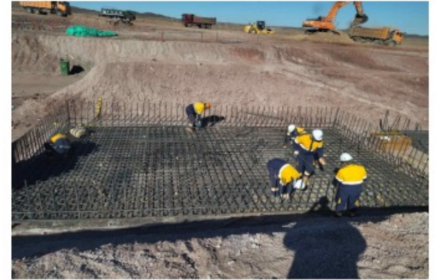
Foundation Rebar Installation
