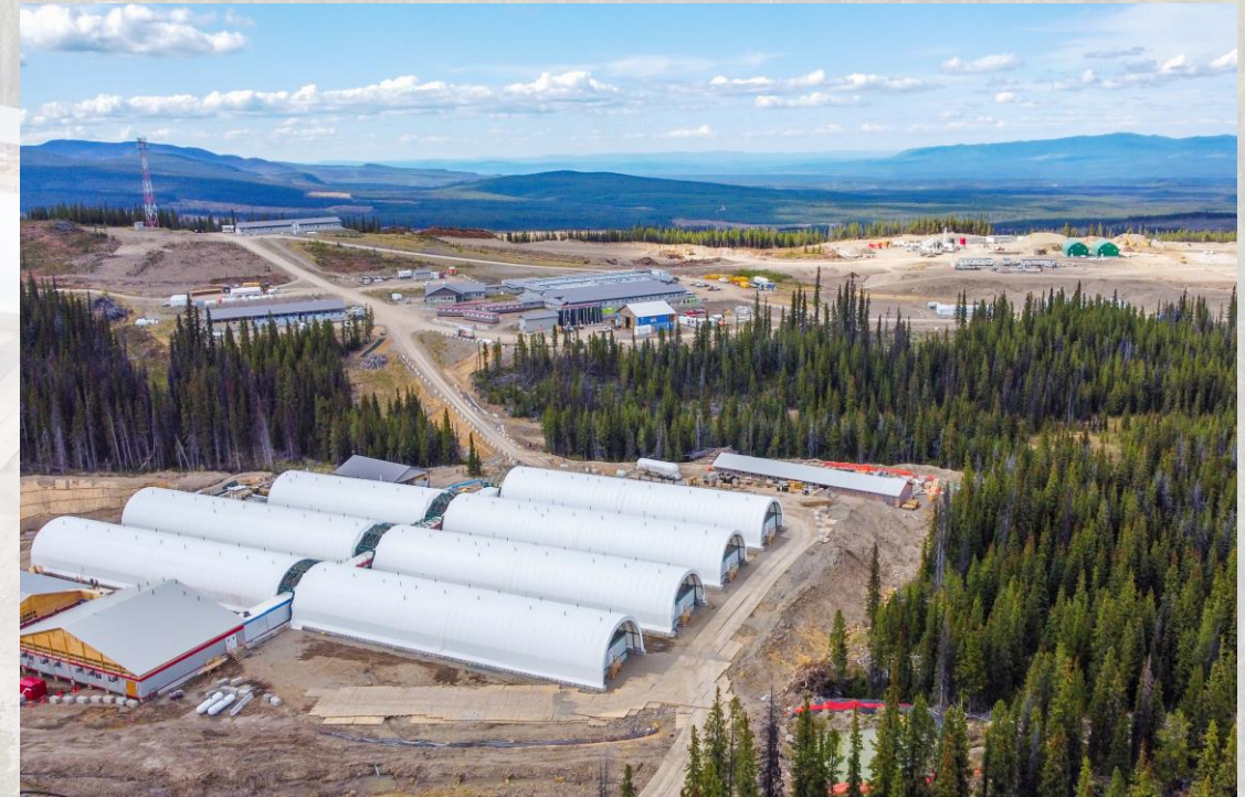
Blackwater Project new construction camp – June 2023
