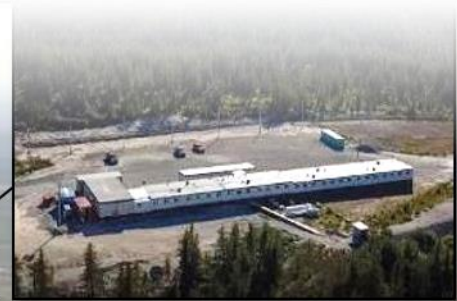
Initial Construction Starter Camp *installed septic
