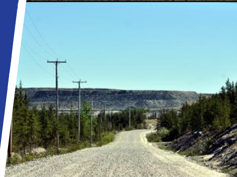
60 km Power Line, Site Roads and River Crossings
