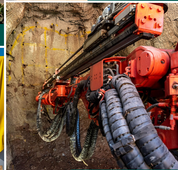
Mine development advances at Portal 2 & 4
