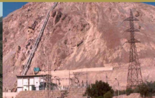
HIGH TENSION POWER LINES
