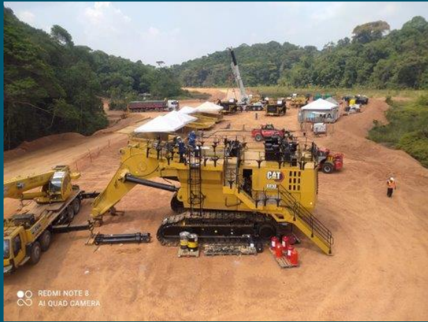
Equipment assembly pad
