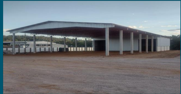
Morais Almeida Logistics Base Complete and Operational
