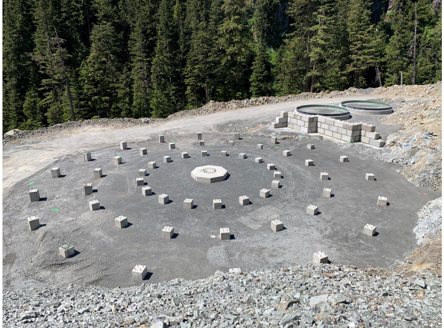
Clarifier and lime silo foundations
