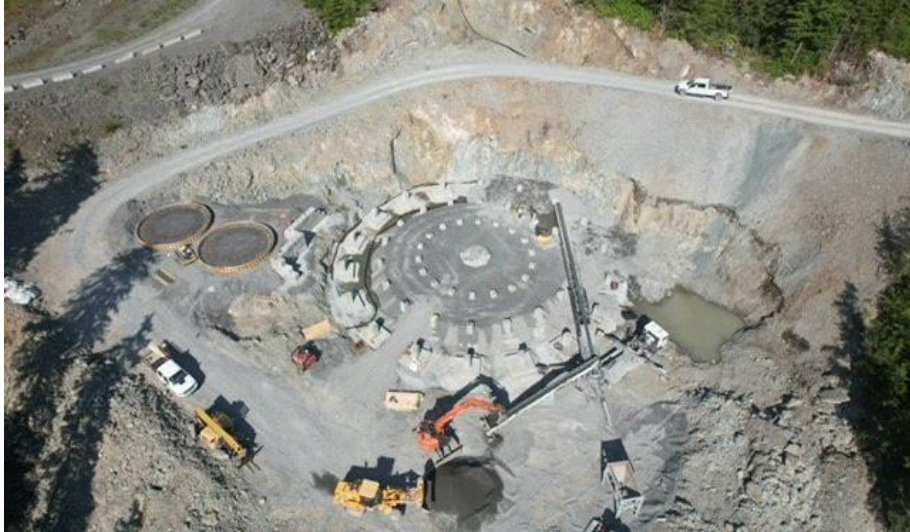
Clarifier foundation and MBBR tank
