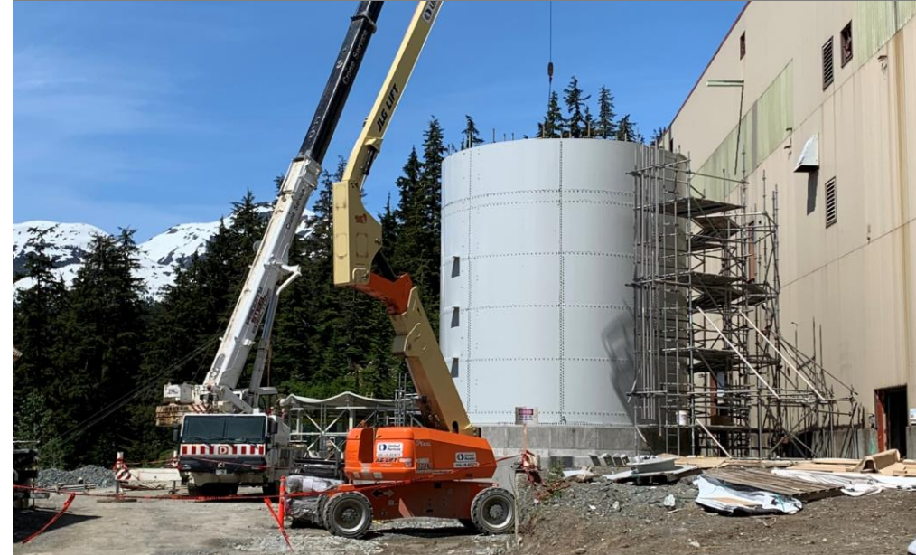
Thickener and CN destruct tank erection
