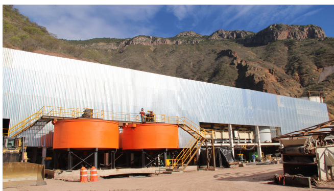
Thickener tanks installed and mill in final stages of assembly
