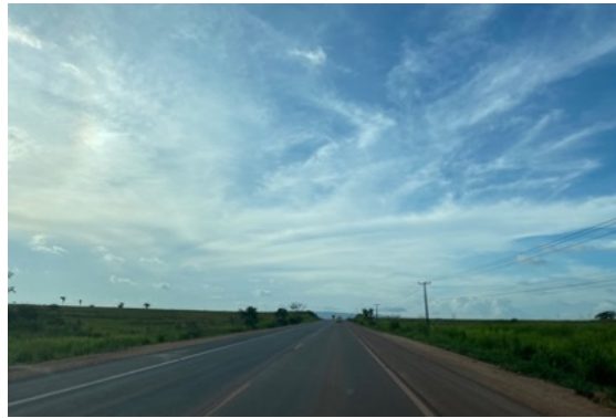
Paved Highway to Site Turnoff
