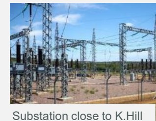
Substation close to K.Hill
