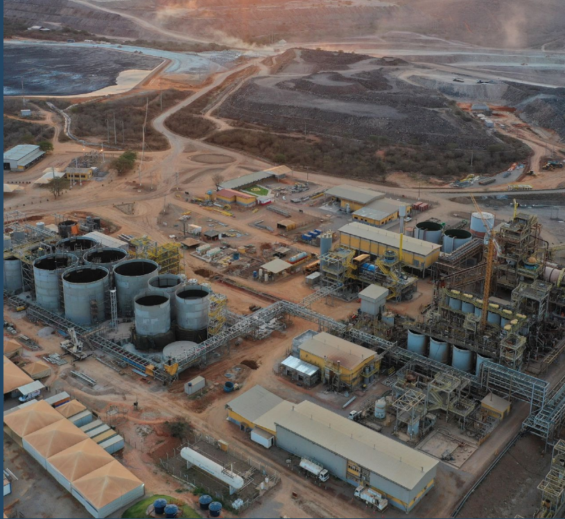
Leach tanks (left), Ball and SAG mill (right) – October 15, 2021
