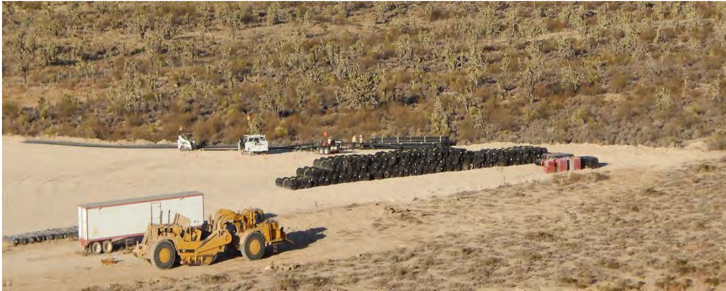
Installing heap leach pad liners
