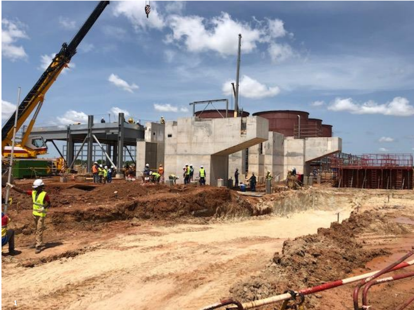
1 Ball and SAG mill foundations
