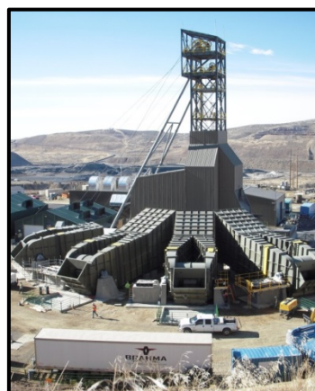
Turf Vent Shaft
