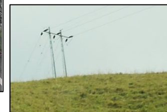
Electrical transmission lines nearby project
