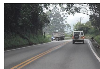
Paved road to project
