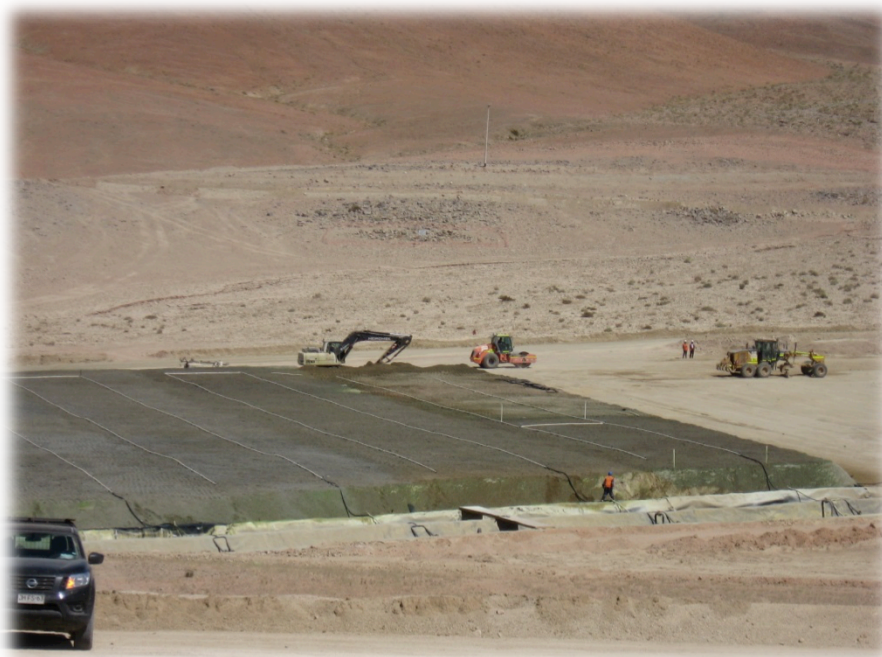
Heap Leaching pads in Berta
