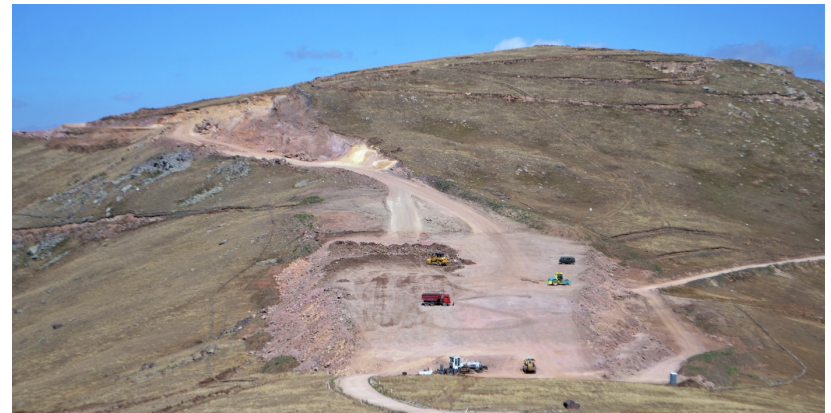
Construction of mine haul road.
