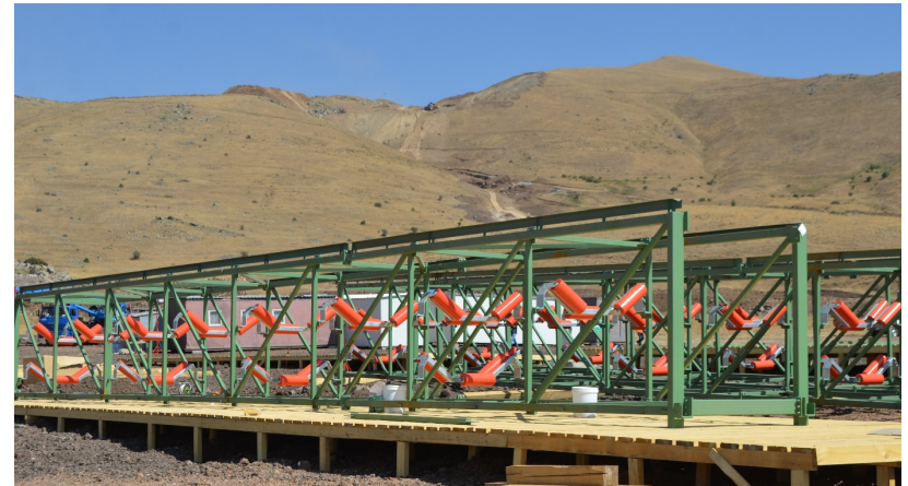
Assembly of conveyor galleries.
