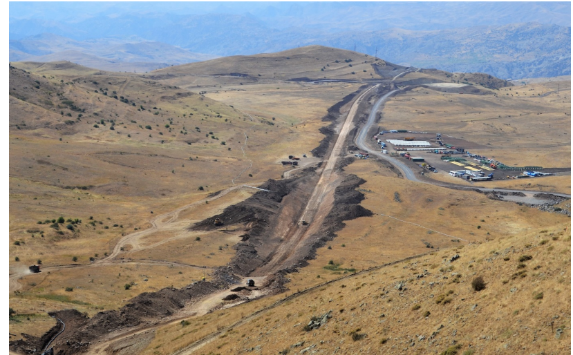
Earthworks for conveyor corridor.
