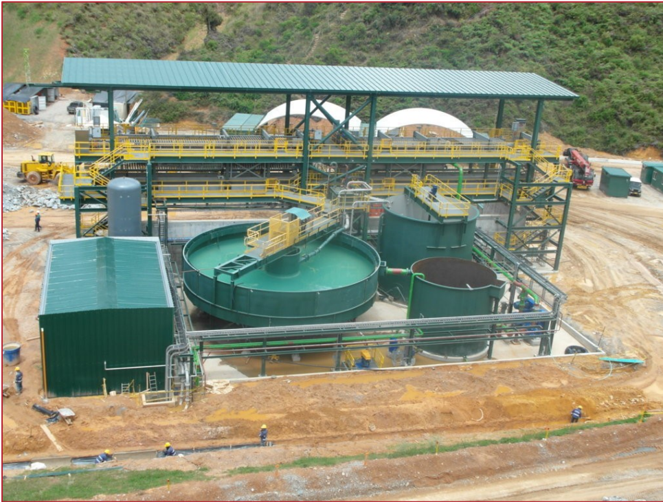
Filter Presses and Tails Area Wet Commissioning
