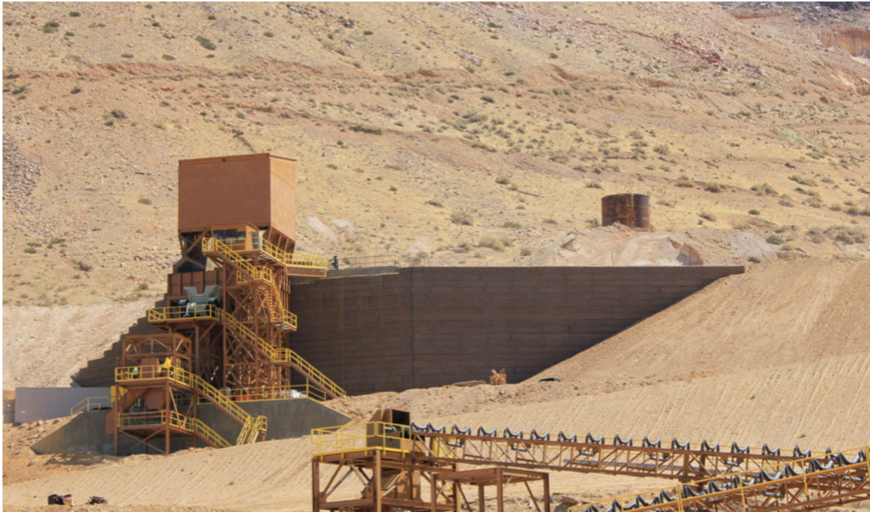
Primary crusher structure
