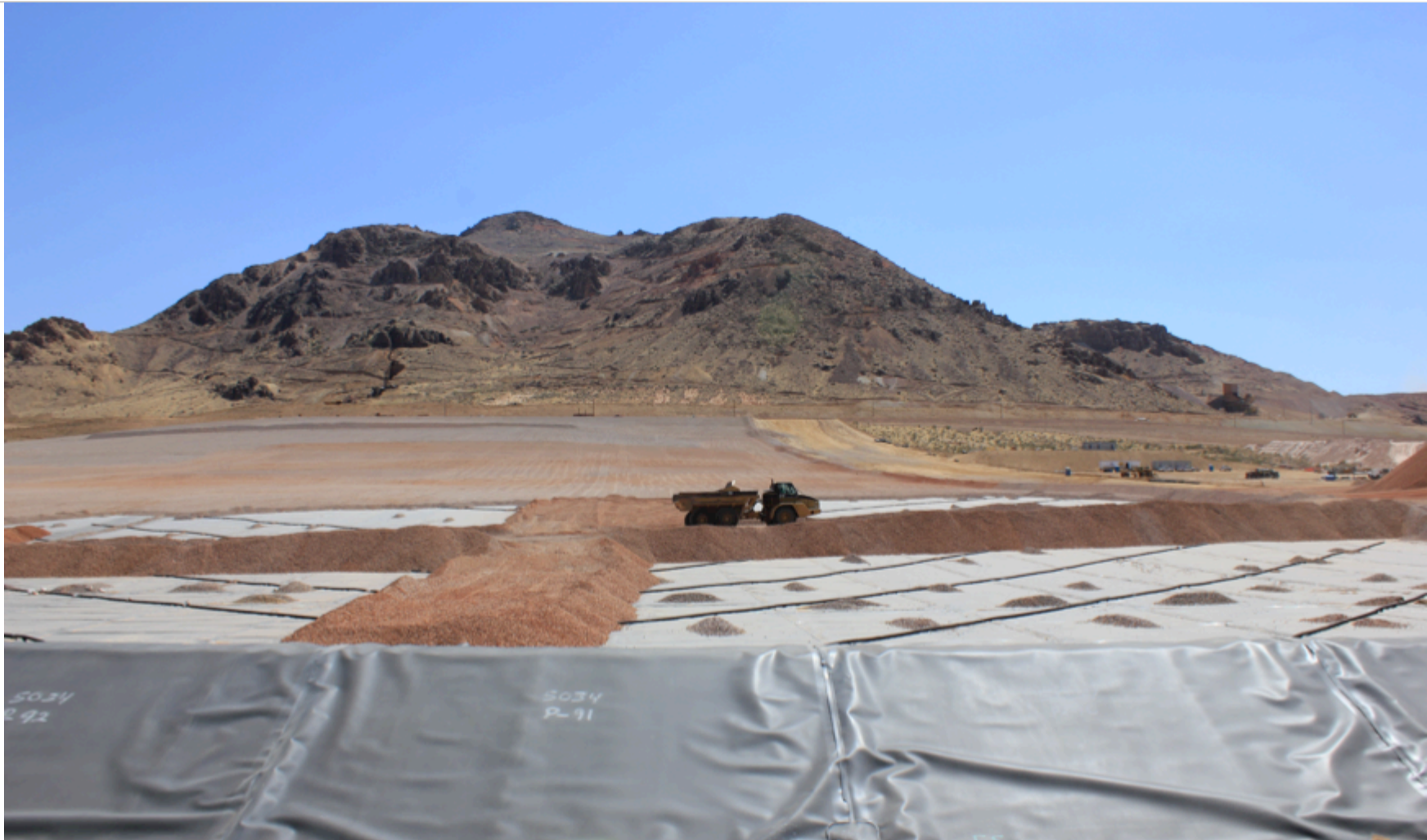
Installation of the heap leach pad overliner
