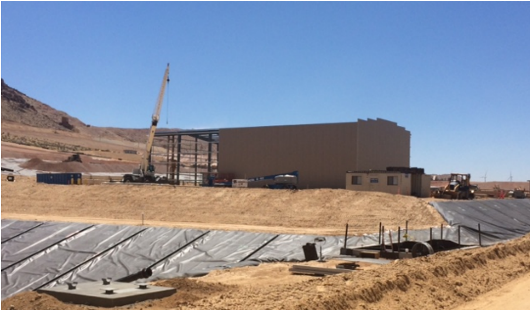
Erection of Merrill-Crowe plant building
