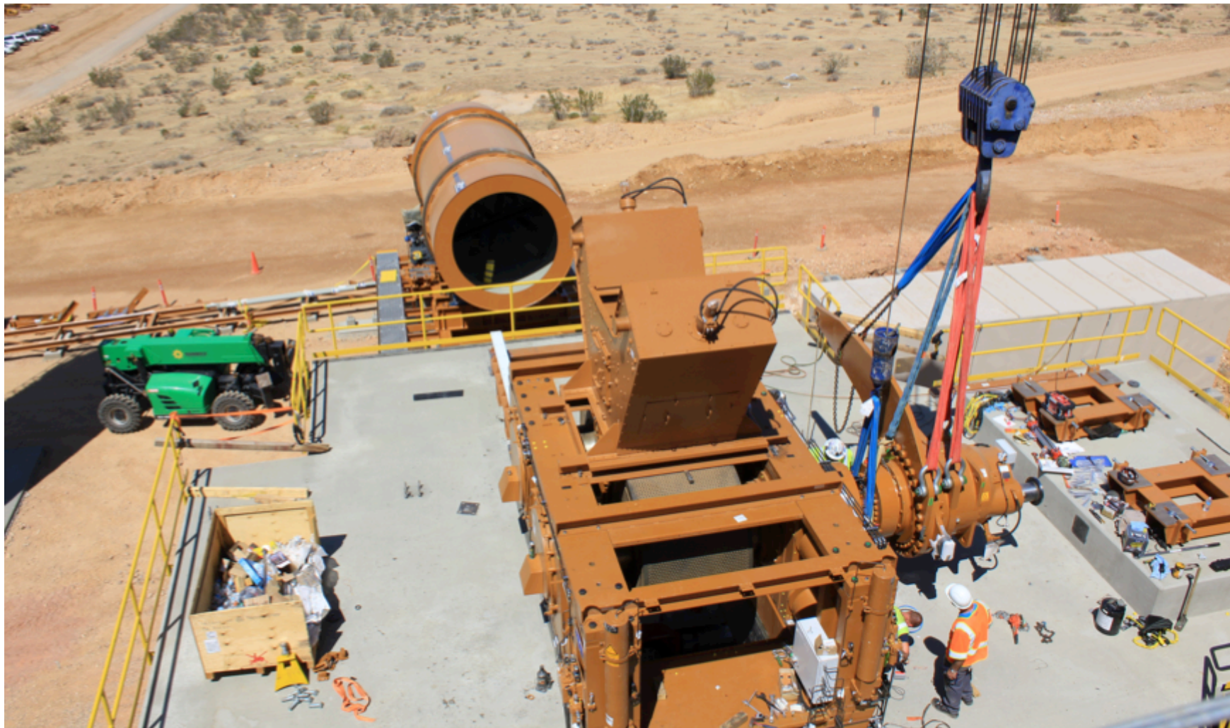
Tertiary crusher structure - HPGR and agglomeration drum
