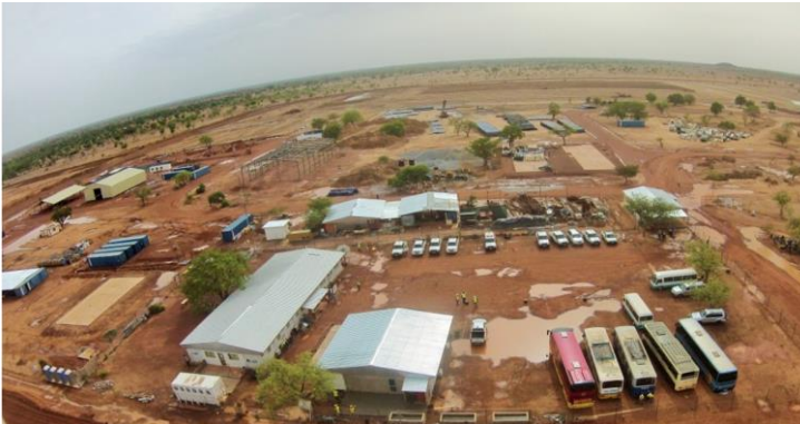
Plant site with offices in foreground, reagent storage buildings on left, maintenance yard top right, and laydown yard centre.
