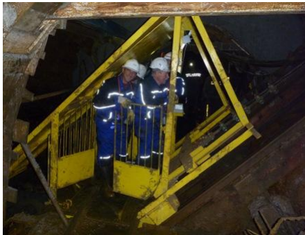
Incline shaft rehabilitated, access from surface to level 6
