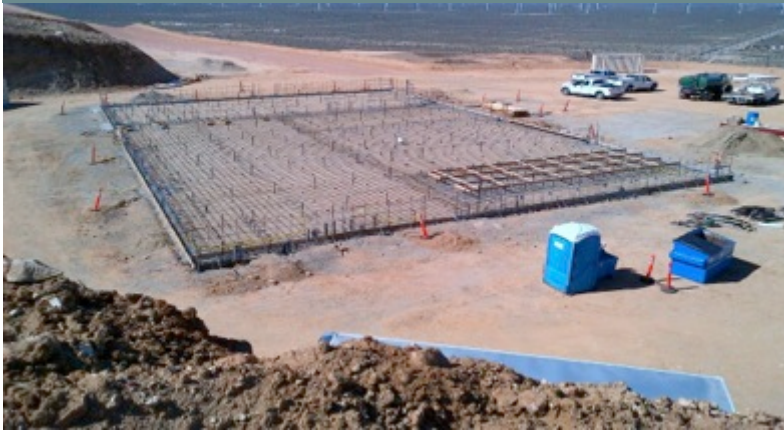
Slab reinforcing steel in place (March 2014)
