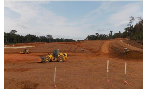
Plant Site - Concrete Batch Plant
