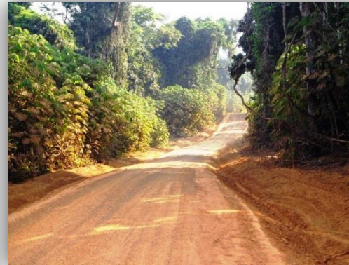
New Laterite Road (20km)
