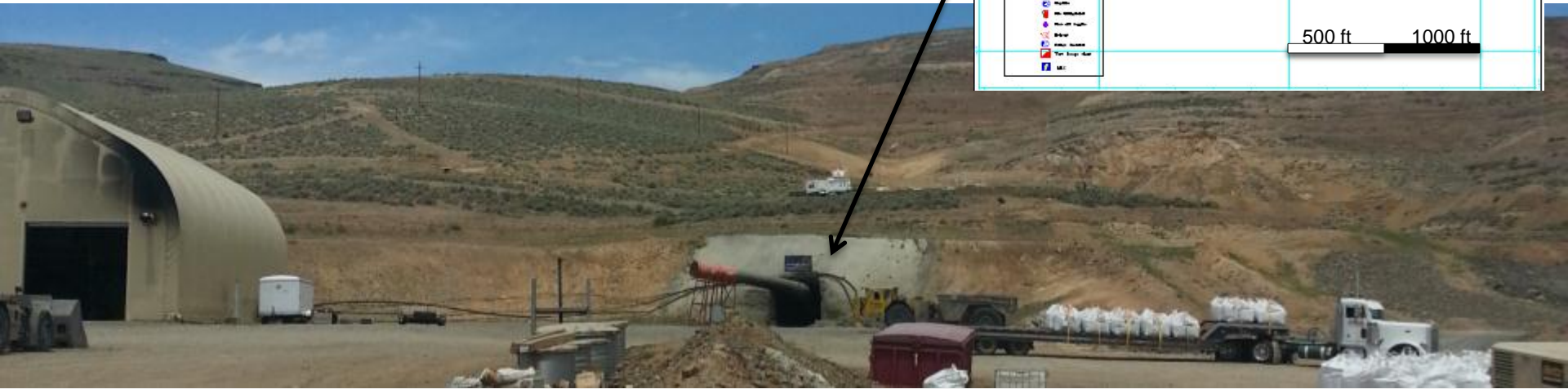
Fire Creek onsite infrastructure: buildings, power line, portal and bags of mineralized material
