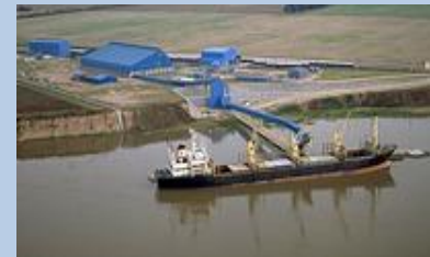
Treatment Facility / Concentrator
