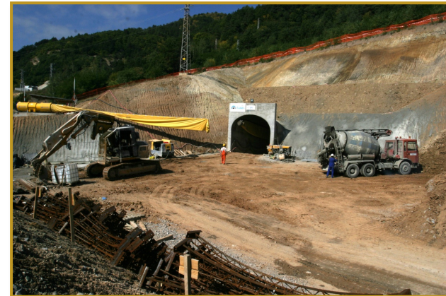
Vyara Portal Construction
