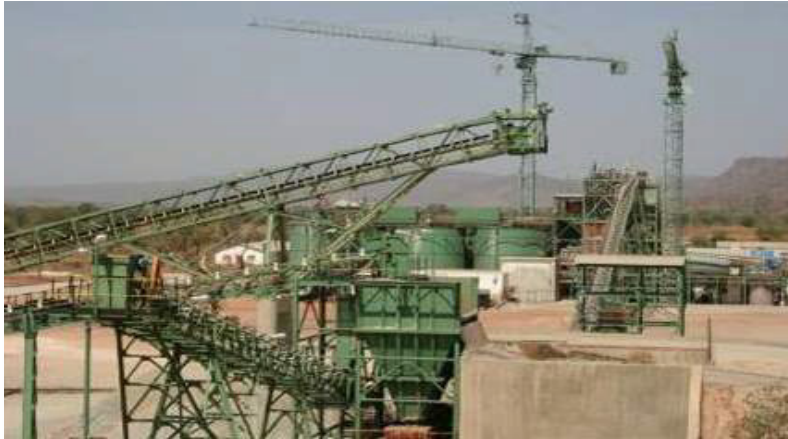
Milling Facility – 2,100 tpd
