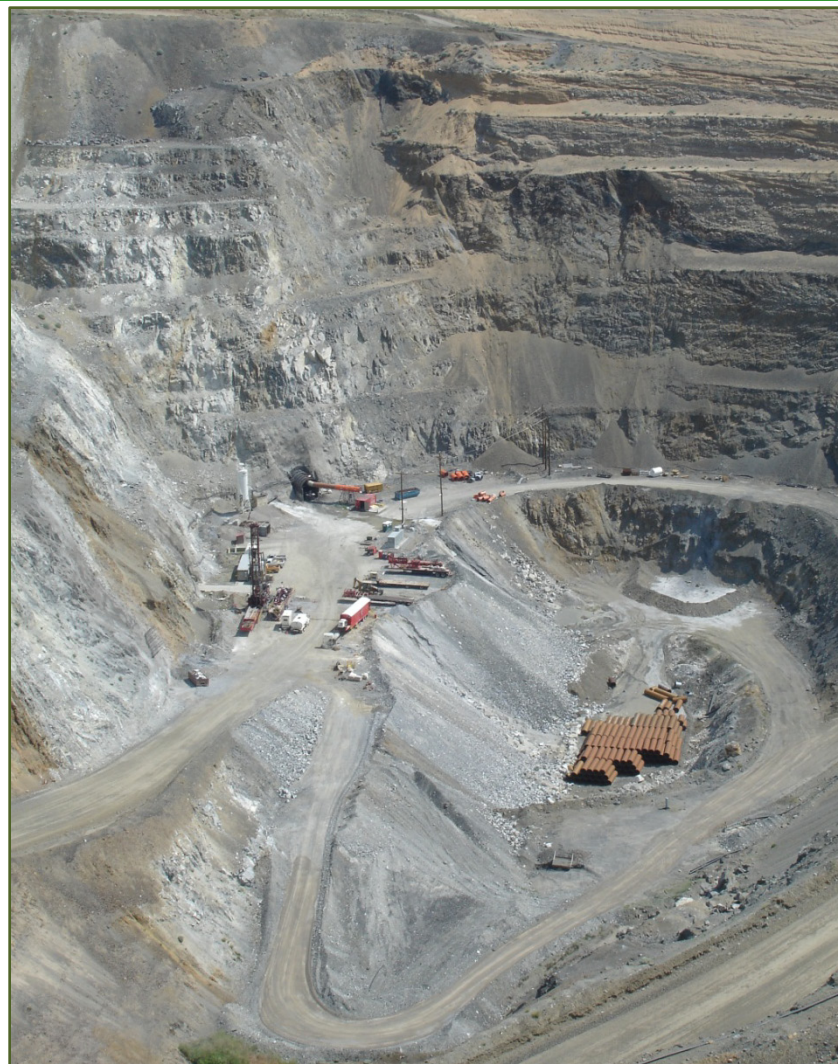
In- Pit Infrastructure
