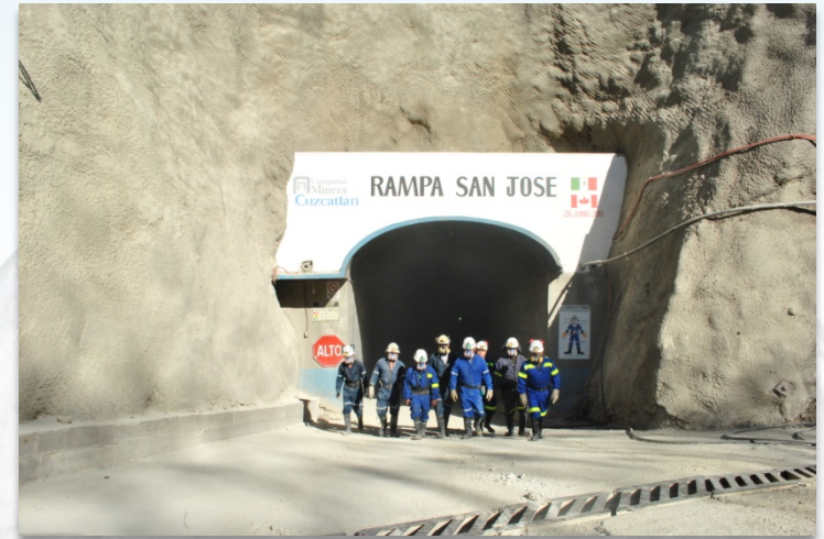
Main access ramp portal
