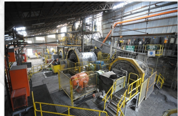
CAYLLOMA MINE: 1,250 tpd processing plant
